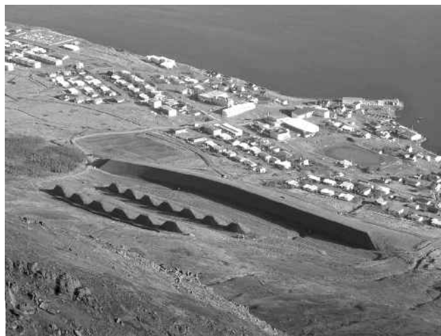
Fig. 1. A photograph of the braking mounds in Neskaupstaður and the catching dam behind them. Each mound is 10 m high, and the catching dam 17 m high.
